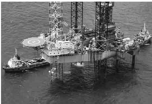
Figure 2 — General view of the offshore oil platform, which used steel piles with aluminum coatings
